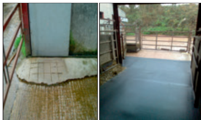
Before: Lumpy Concrete After: Rubber Matting
