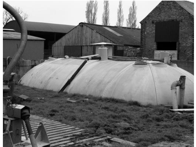
Small anaerobic digester on Trevor Lea's organic dairy farm in Wales. The biogas is used to supply hot water to the milking parlour, dairy and farmhouse.
