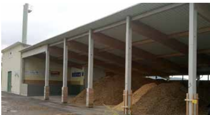
Wood-chip drying undercover before use in the Oberrospe burner to provide heat for 55% of the town's households
